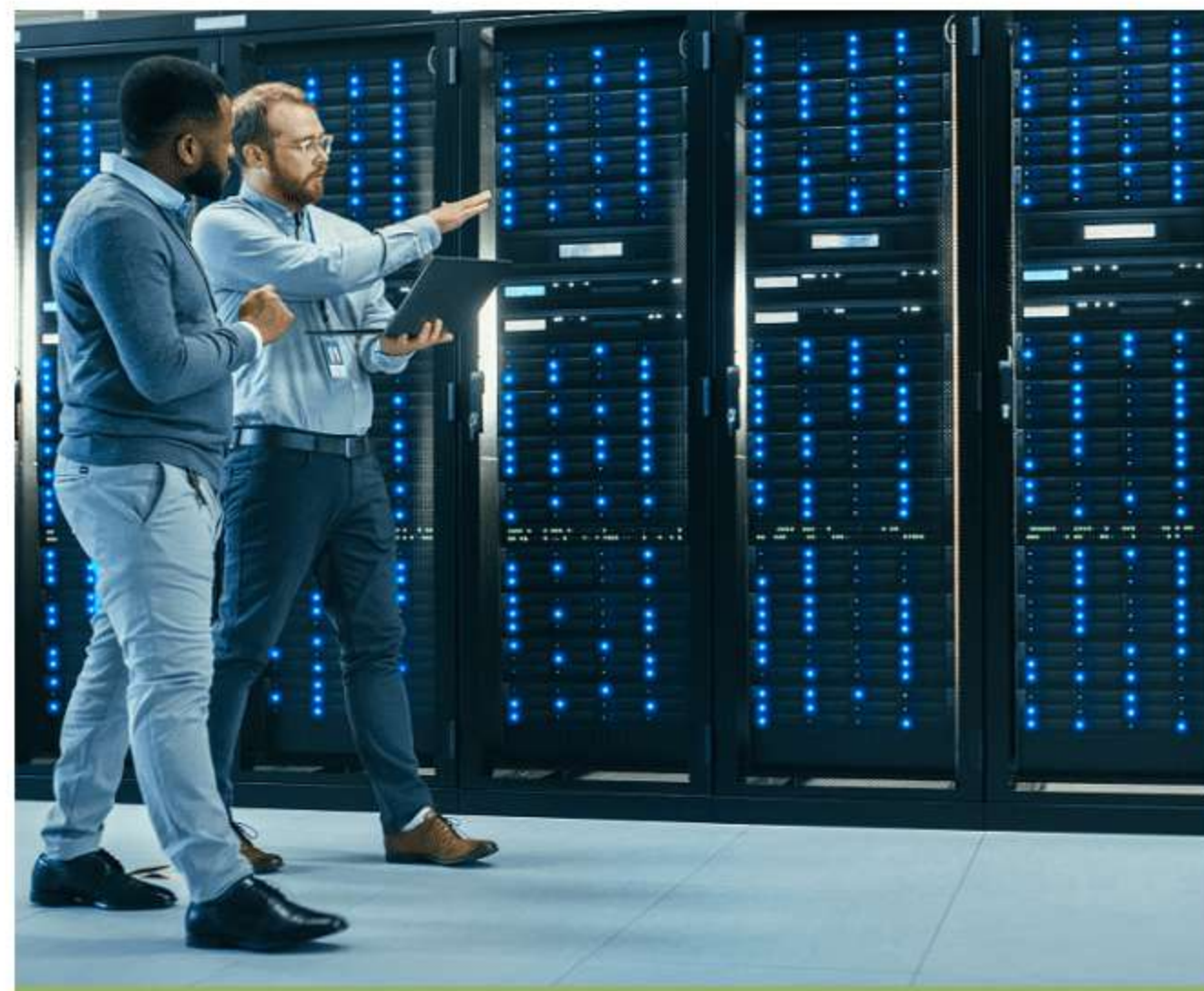
DATA CENTRE SOLUTION
